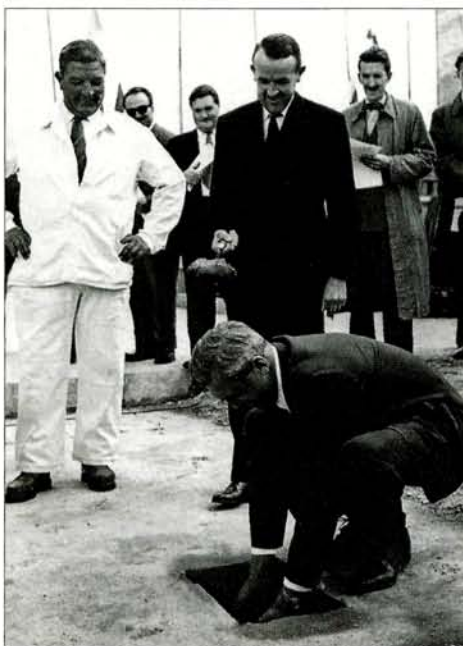
The foundation stone was laid on 10 June 1952 in the presence of Swiss and CERN authorities. Felix Bloch, CERN's first director-general, laid the stone on the laboratory site, watched by Max Petitpierre, then president of the Swiss Confederation.
