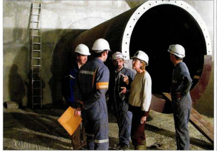
Natacha Lopez (centre), the engineer at CERN in charge of contracts for the design and construction of the decay tube, with some of the team near, literally, the end of the project.
