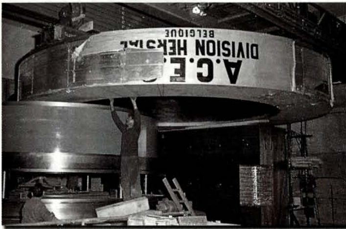
The upper magnet coil of CERN's first machine, the Synchrocyclotron (SC), is moved over the upper pole discs. Each coil weighed 60 tonnes and measured 7.2 metres in diameter. The SC was commissioned in 1957 and was operational for 34 years.
