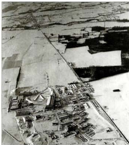
While taking this aerial view in 1963, Roger Anthoine – who was also at the controls of the aeroplane – braved a temperature of -25^{\circ}\text{C} .
